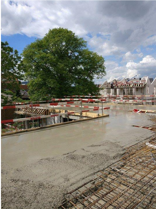
PICTURE 12. Pouring concrete
