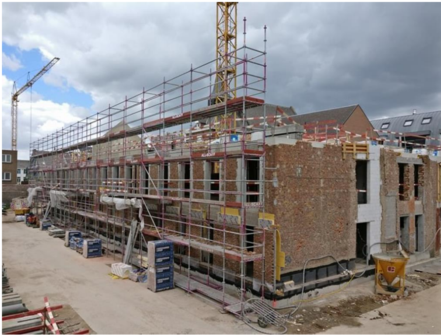
PICTURE 7. Renovation of the pre-existing building in June 2017.
