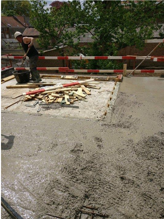
PICTURE 11. Situ concrete of this detail
