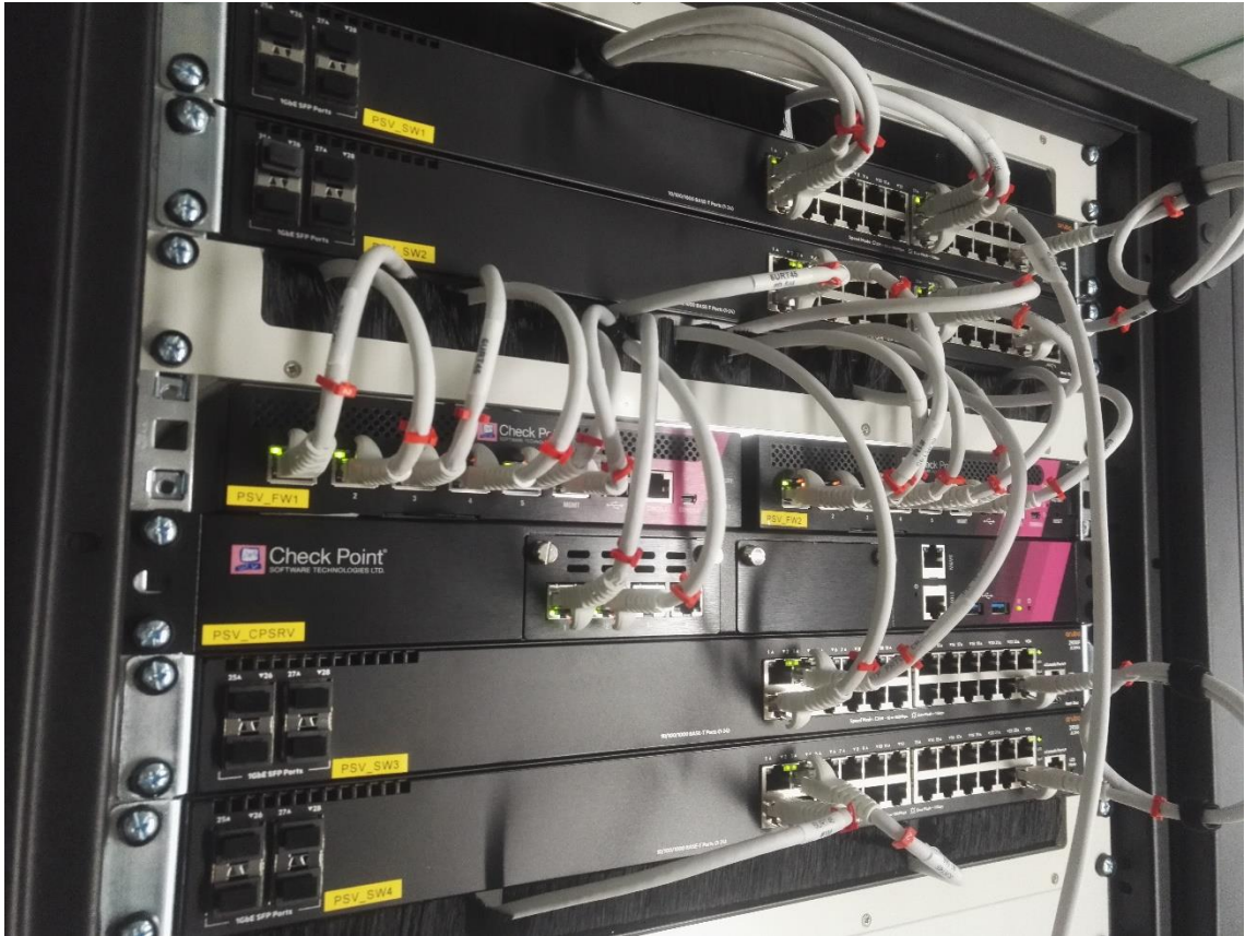
Picture 21. Finished Cluster installation.
