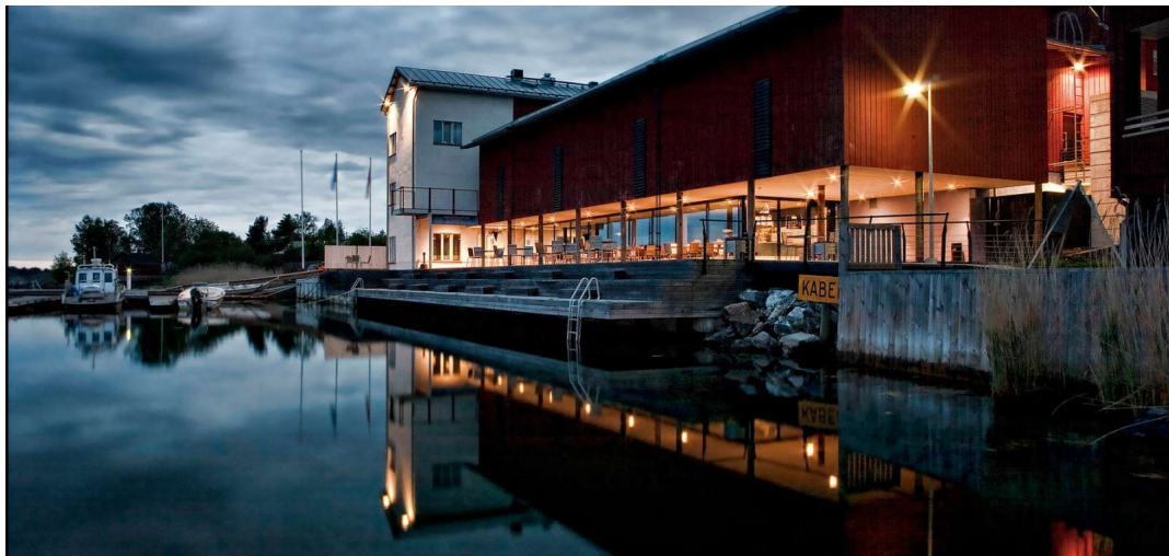
Picture 5. The main building and the terrace. (Jansson 2017.)
