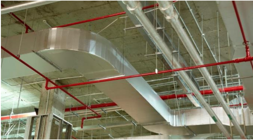
Figure 4.9. Rectangular ductwork
