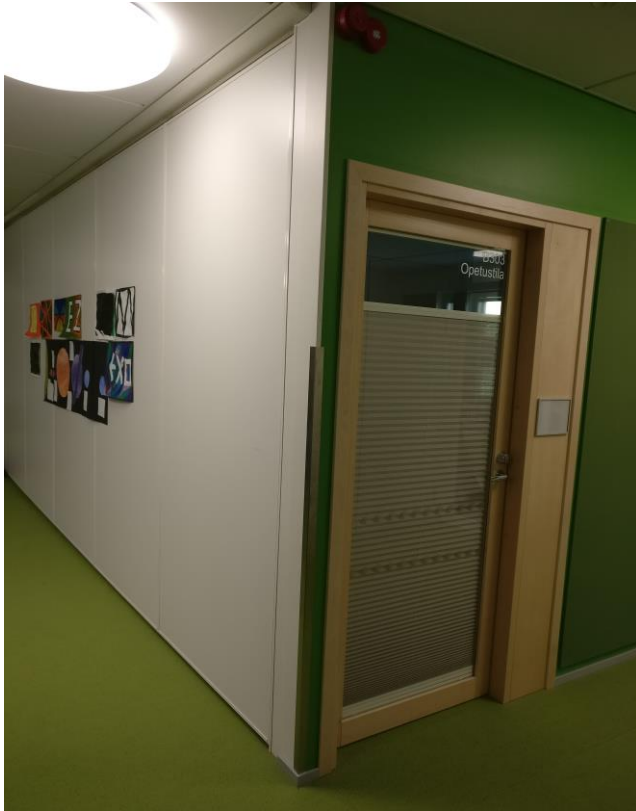
Figure 6.6. Some of the walls are movable (the white wall in the picture)
