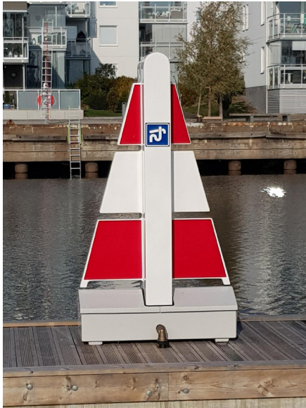
Pictures 10a, 10b. Municipality sewage connected septic waste pump-out station in Gävle city port. © Marita Olsson Narving
