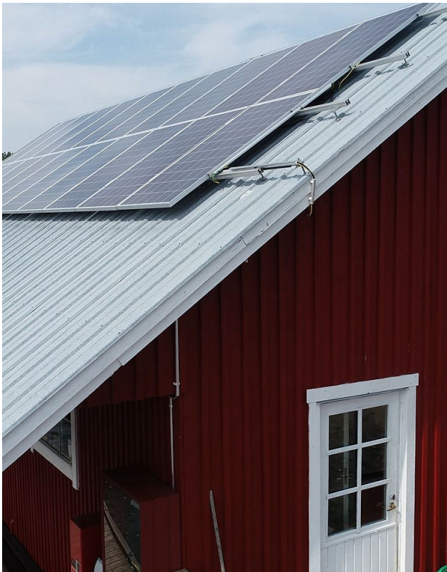
Picture 7. PV system installation. Panels attached parallel to roof and wiring goes from roof to solar inverter via shortest route to protecting custom-made inverter casing on the wall. © Kristiina Kortelainen
