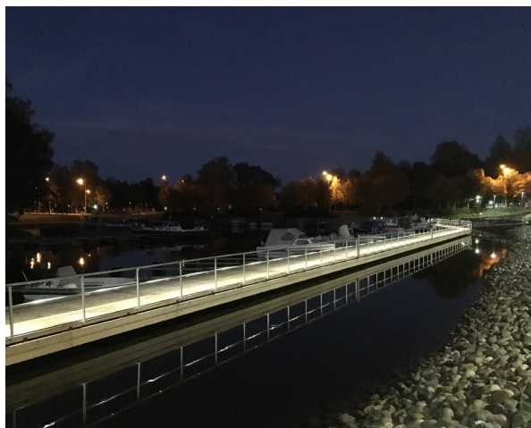
Picture 2b. Dock LED lighting in Syväraumanlahti, Rauma. © Markus Savolainen
