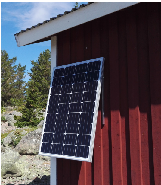
Picture 6. PV panel installation example where upper part of panel is shaded during noon in June. © Kristiina Kortelainen
