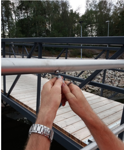
Picture 3. Installation of dock LED lighting ongoing in Syväraumanlahti Rauma. © Markus Savolainen
