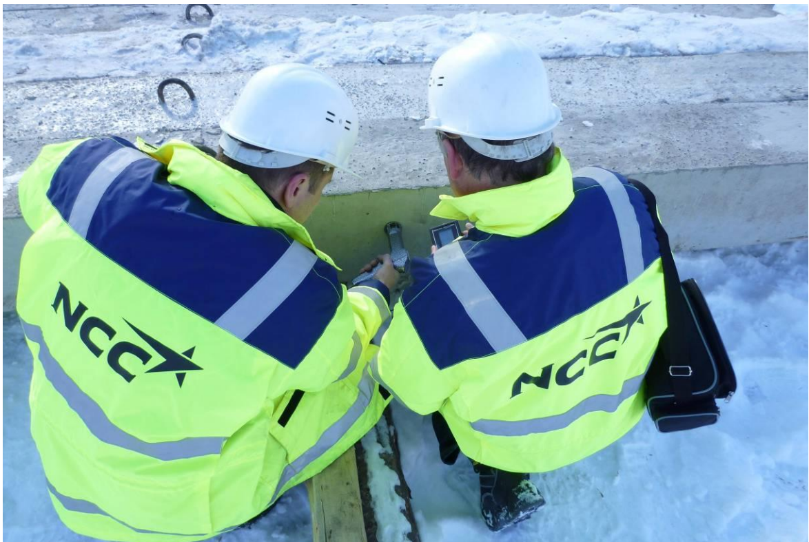
Figure 19. Measuring of the concrete strength at the site
