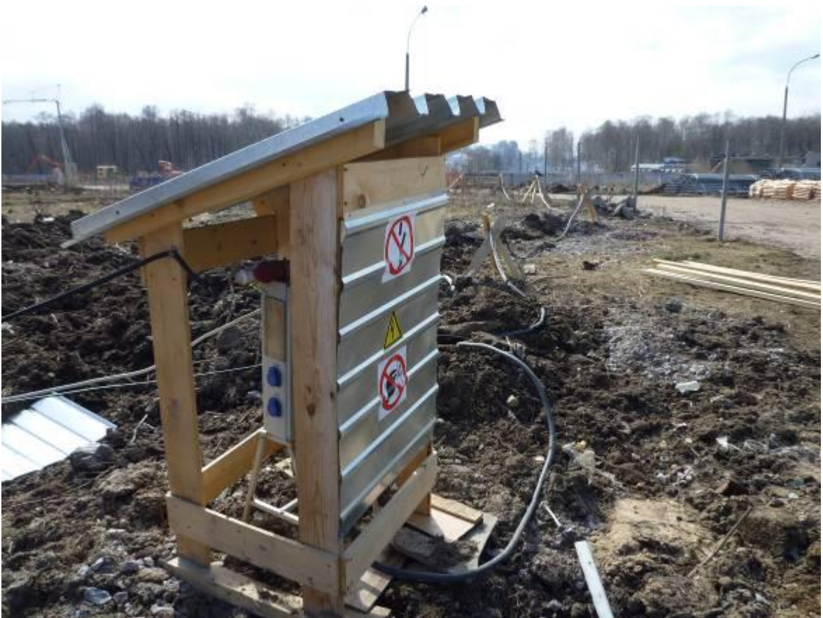
Figure 5. Cable laying and electrical board protection
