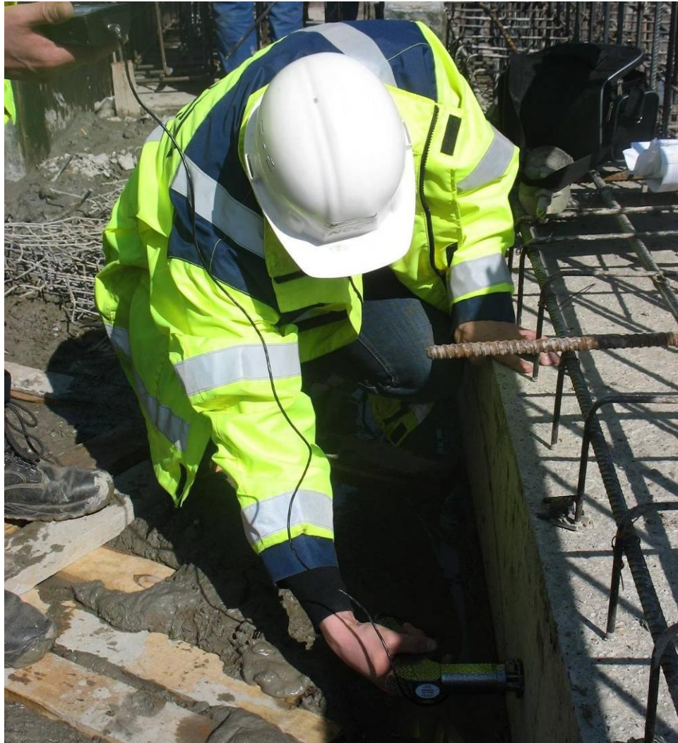
Figure 23. Casted concrete strength measuring
