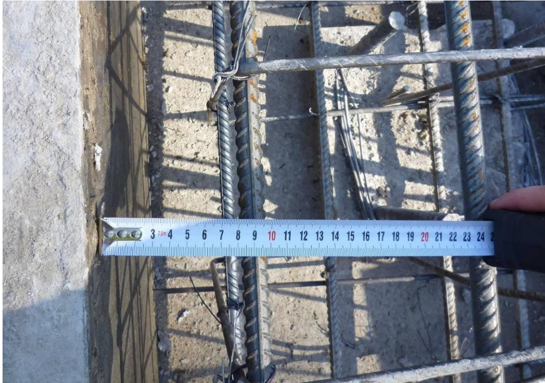
Figure 24. Control of the thickness of the concrete protective layer
