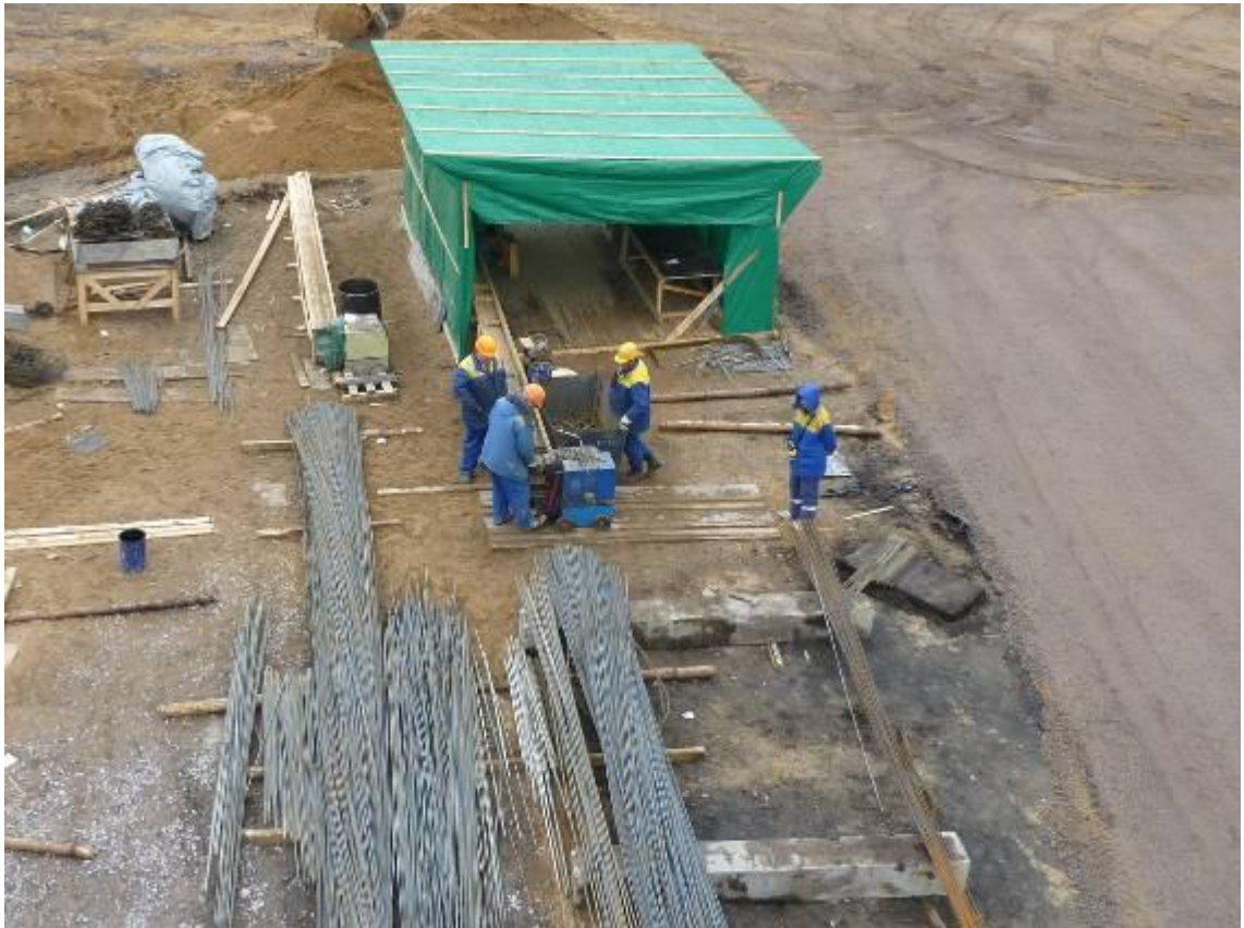
Figure 12. Reinforcing steel shop on a building site
