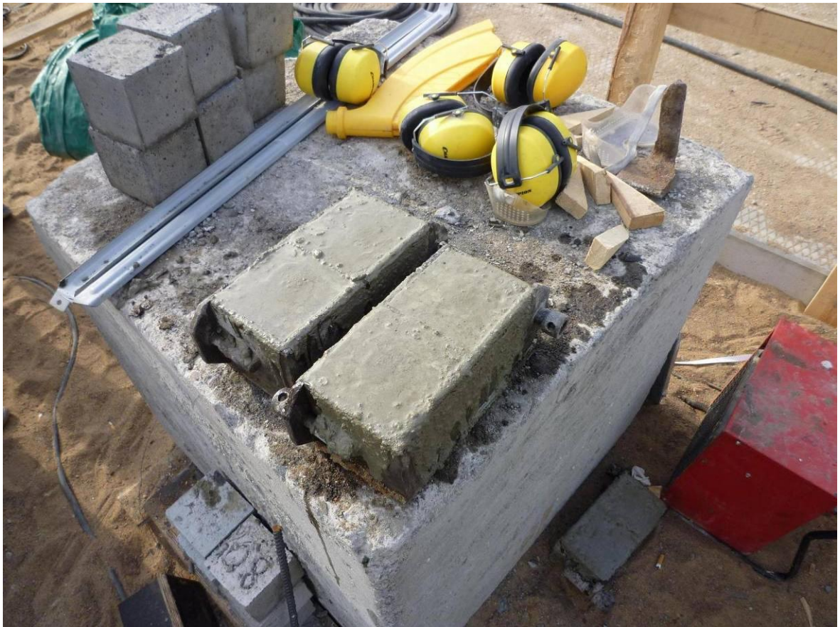
Figure 22. Manufacturing of concrete blocks for the strength tests
