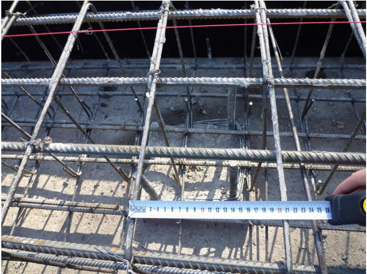
Figure 25. Controlling measurements of rebar spacing in a cage
