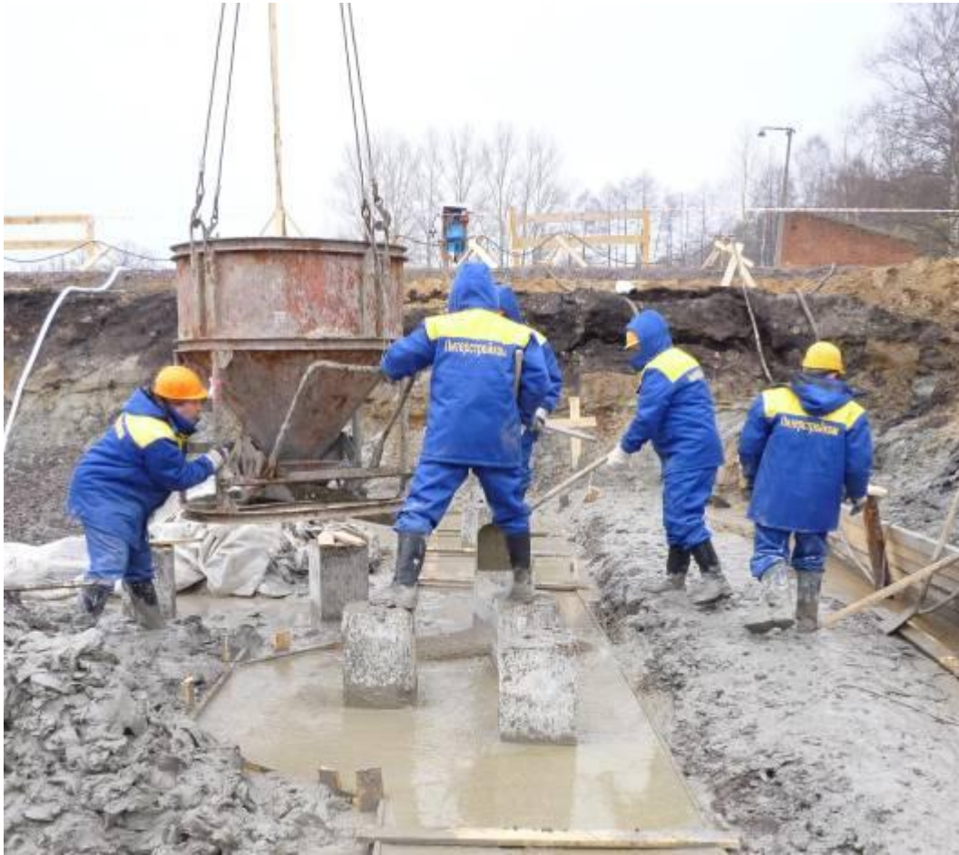
Figure13. Feeding of concrete through the bunker
