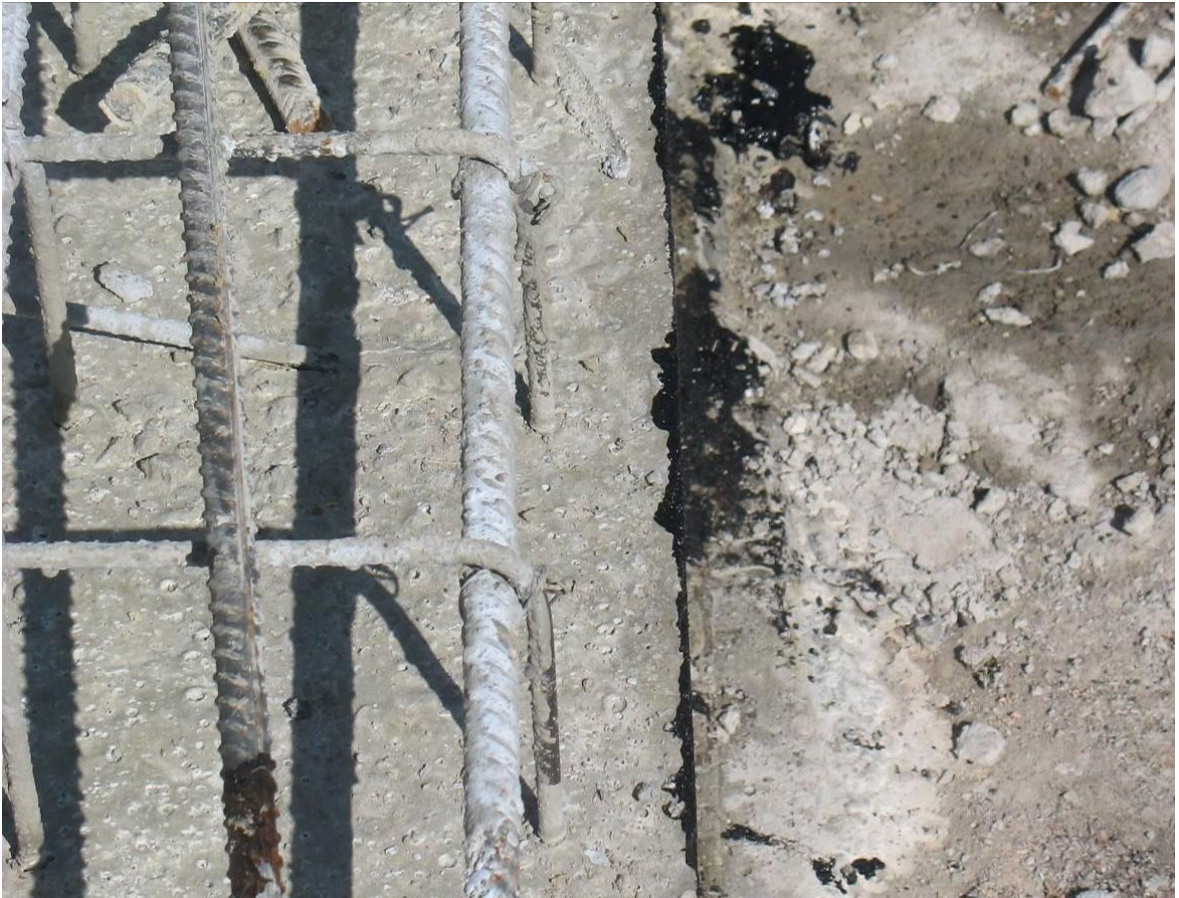
Figure 26. Concrete protective layer after the removal of the formwork
