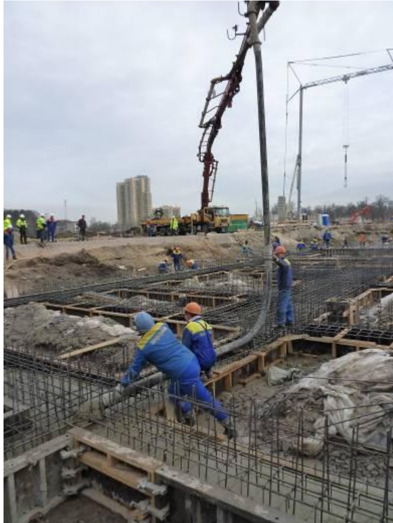
Figure 14. Concreting with the help of a concrete pump
