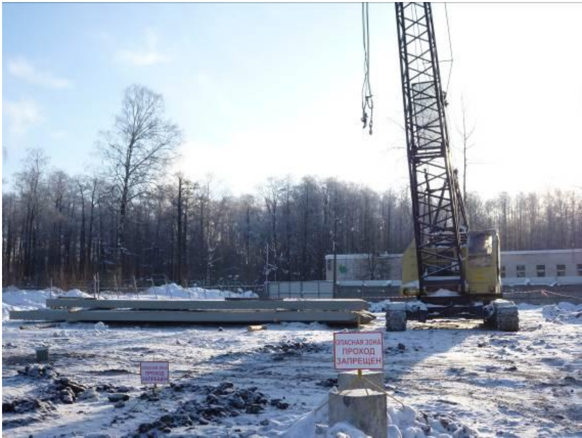
Figure 10. Pile storing area
