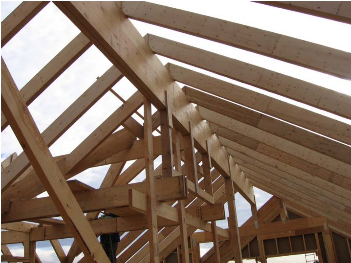
Figure 3.4 Ridge beam (Building materials 2007)
