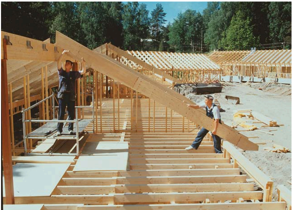
Figure 3.3 Common rafters (FreeTorg 2007)
