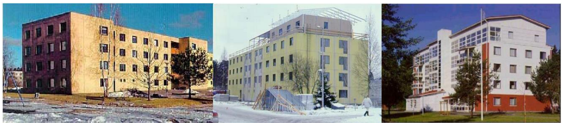
Figure 7. Adding floor reconstruction of a residential building in Finland using lightweight cold rolled sections (Caroli, 2009)
