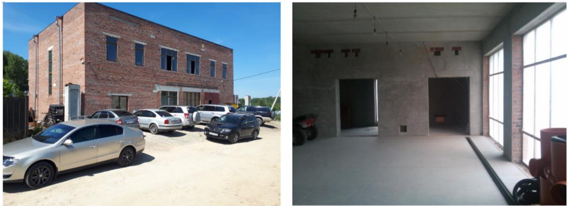
Figure 32. Original building: general view and internal space
