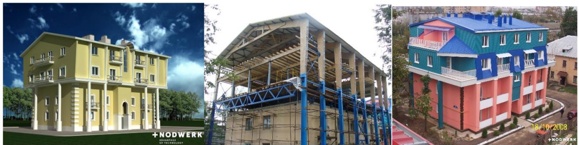
Figure 9. Reconstruction of a two-storey attic in the Republic of Karelia (Nodwerk 2008)
