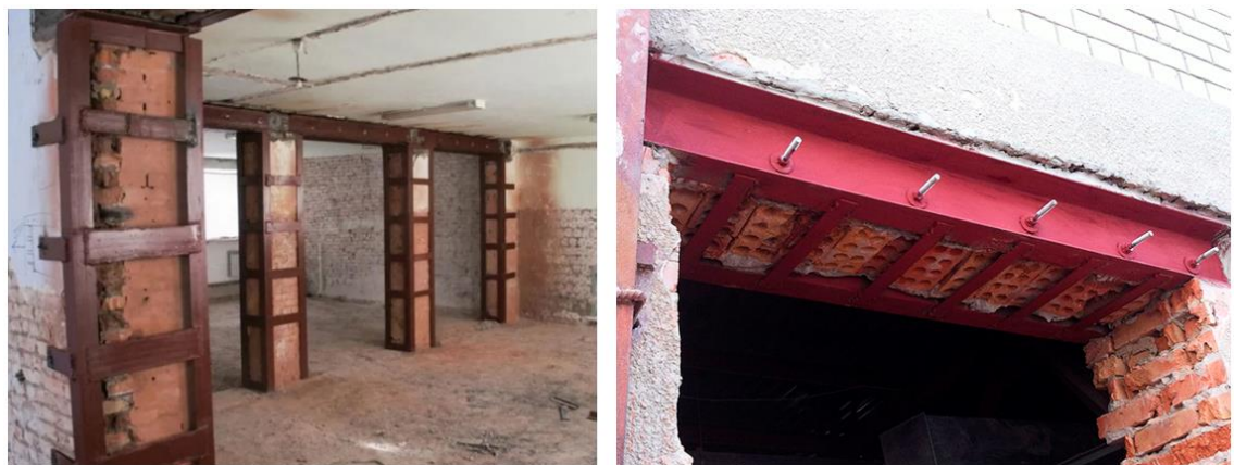
Figure 3. Brick structures strengthening (Almaz-Rezka. n.d.)
