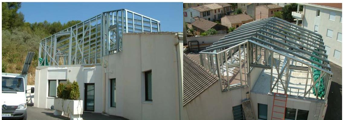
Figure 7. Adding floor reconstruction of a residential building in Finland using lightweight cold rolled sections (Caroli, 2009)
