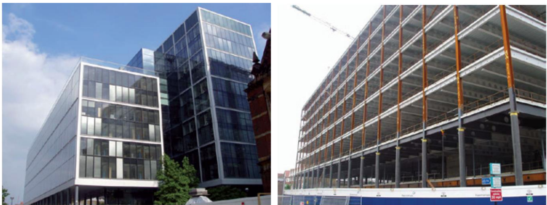
Figure 30. Bishop's Square office building with composite steel-concrete floor (Arcelor Mittal & Peiner Träger 2008 b)
