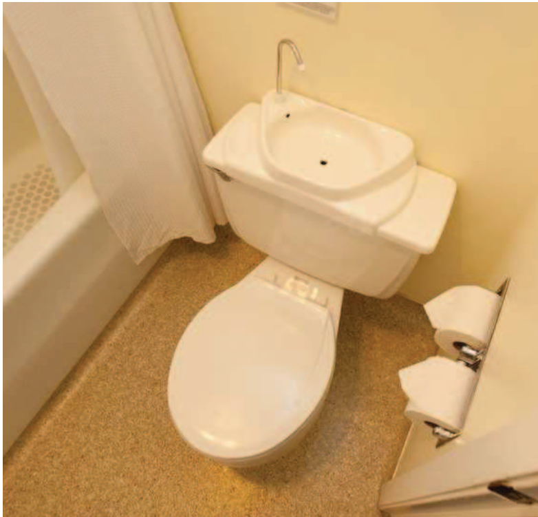
FIGURE 9. Water-saving toilet top sink system. (Oyster Travel Corp 2010)
