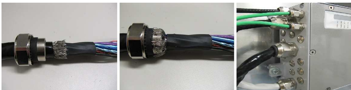
Figure 6. Proper usage of a cable gland in a WTB
