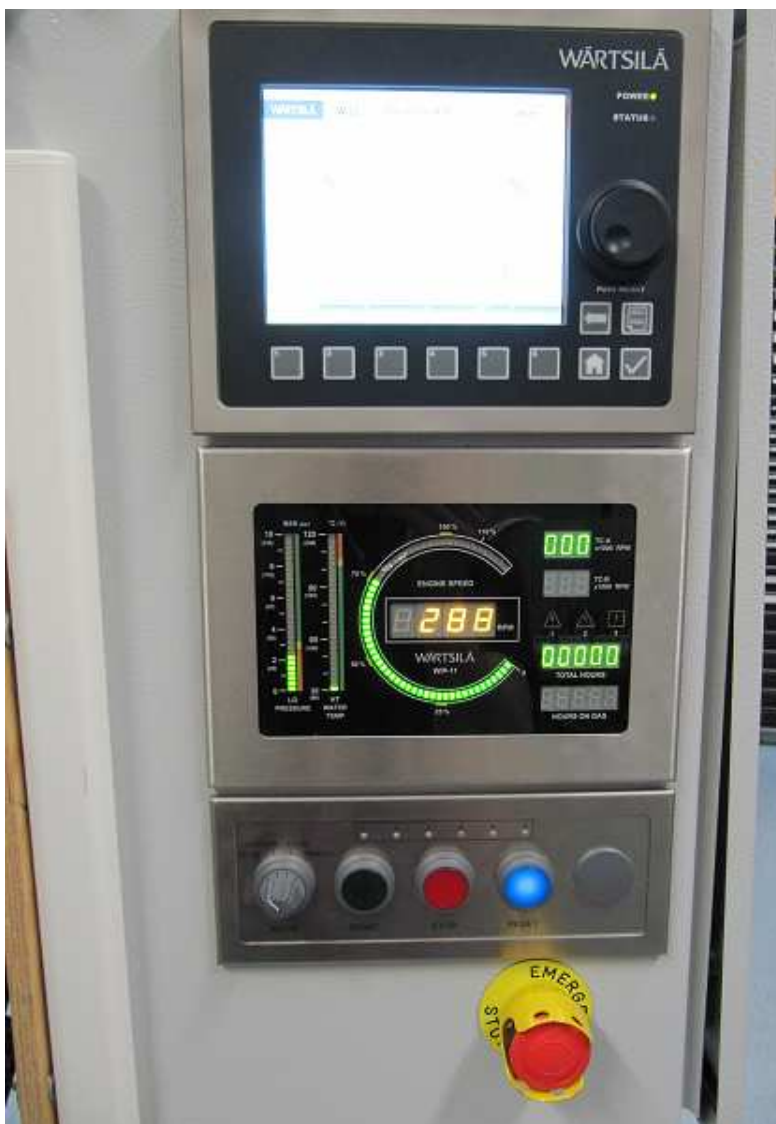
Figure 1. Local Control Panel consisting of a LDU-20, WIP-11 and a WCP-10.
