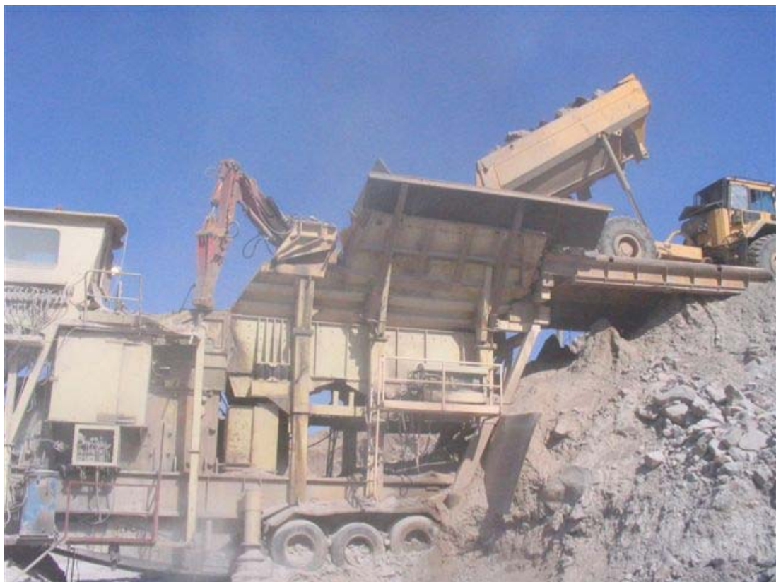
PICTURE 2. Aggregate crusher (NCC Roads)
