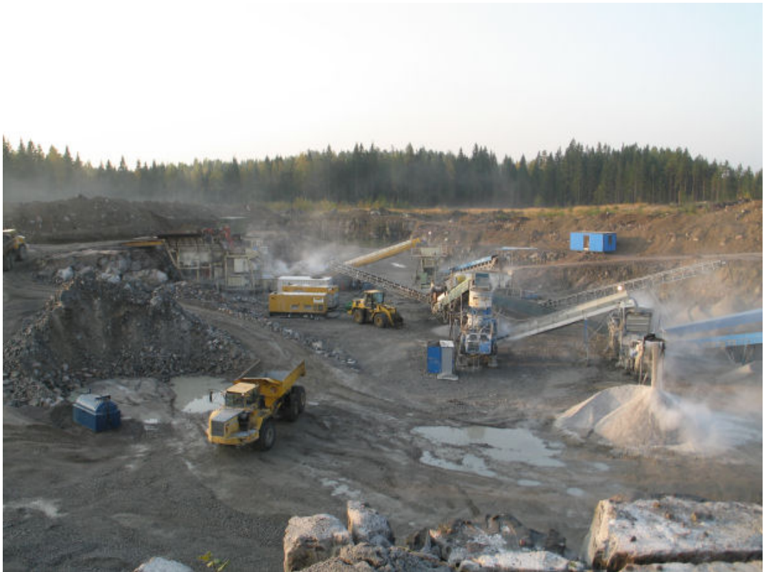
PICTURE 1. Aggregate production site (NCC Roads)
