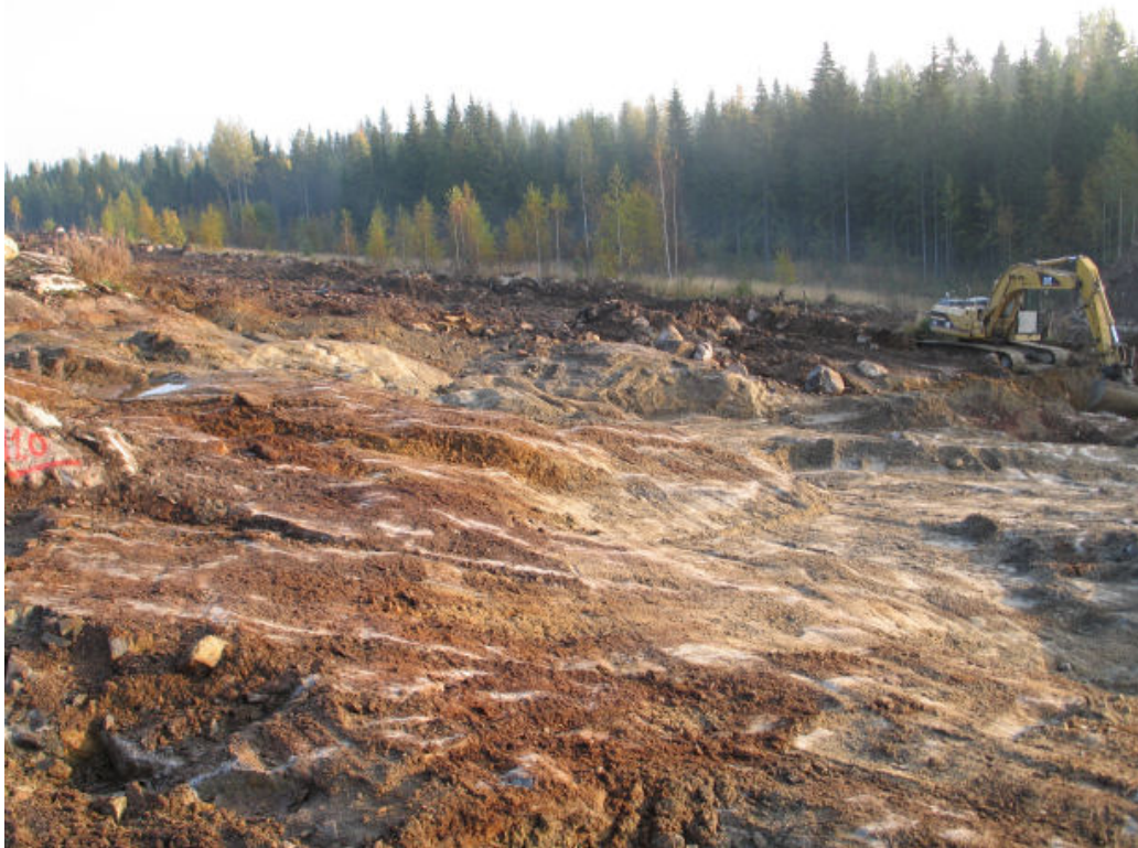
PICTURE 3. Removal of the overburden layer (NCC Roads)
