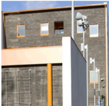
Figure 9: Brick wall, real world photo [20]
