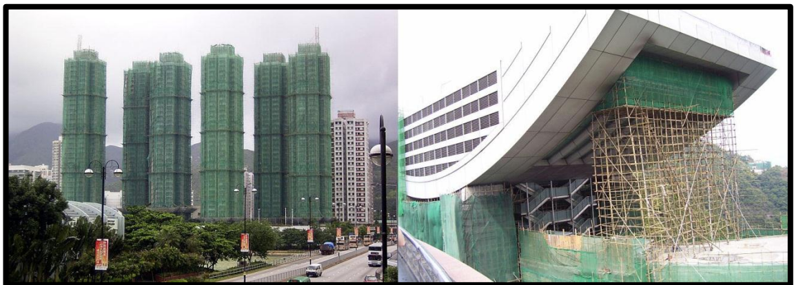
Figure 4 Bamboo high-rise scaffolding in Hong Kong, China
