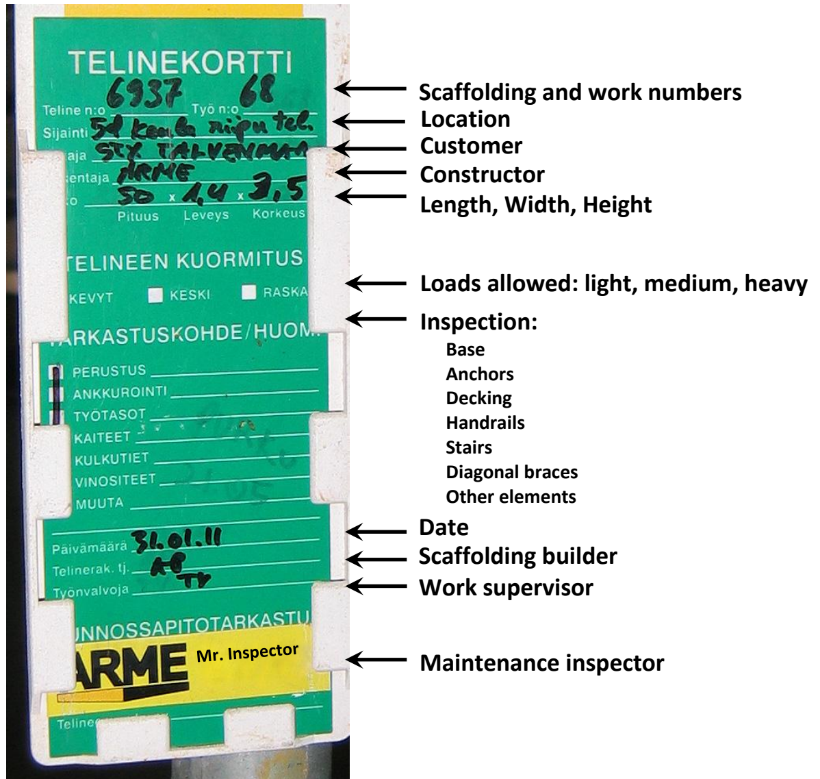
Figure 48 A closer look at the Finnish scaffolding tag
