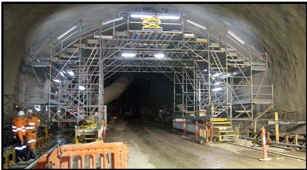
Figure 22 Modular mobile scaffold gantry in the tunnel, Australia
