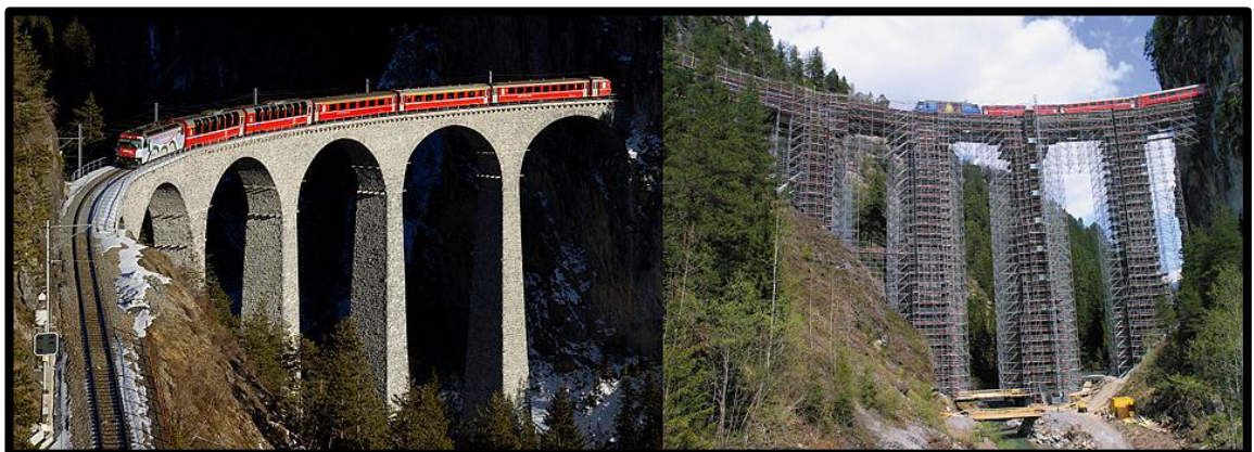
Figure 1 Modular scaffolding - renovation of the Landwasser Viaduct in Switzerland
