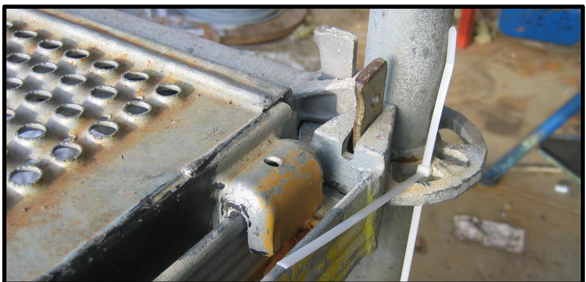
Figure 43 Deck carried by U-shaped transom
