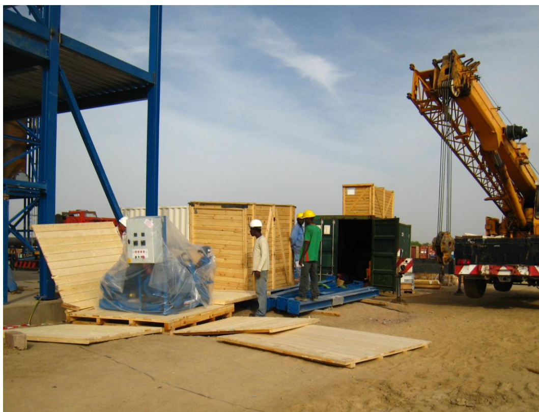
Figure 5. The module is packed in a wooden box and covered with a plastic coating. /17/
