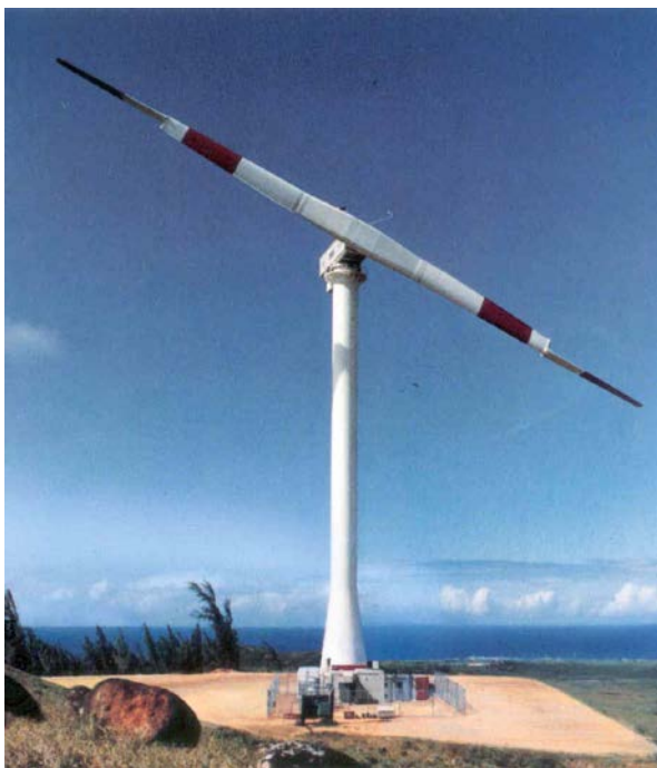
Figure 4. The 98 meter diameter, two-bladed NASA/DOE Mod-5B wind turbine was the largest operating wind turbine in the world in the early 1990s. (Wikipedia: Mod-5B, 2011).
