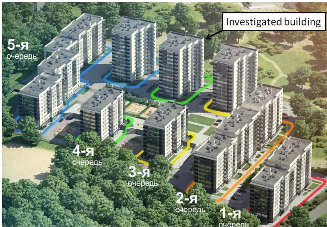
FIGURE 13. Housing estate “Swedish Krona” /19/
