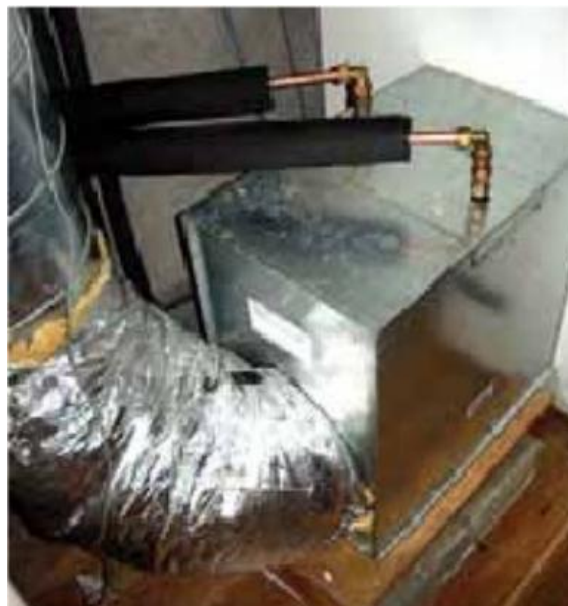
FIGURE 14. Water-to-air heat exchanger unit /2/
