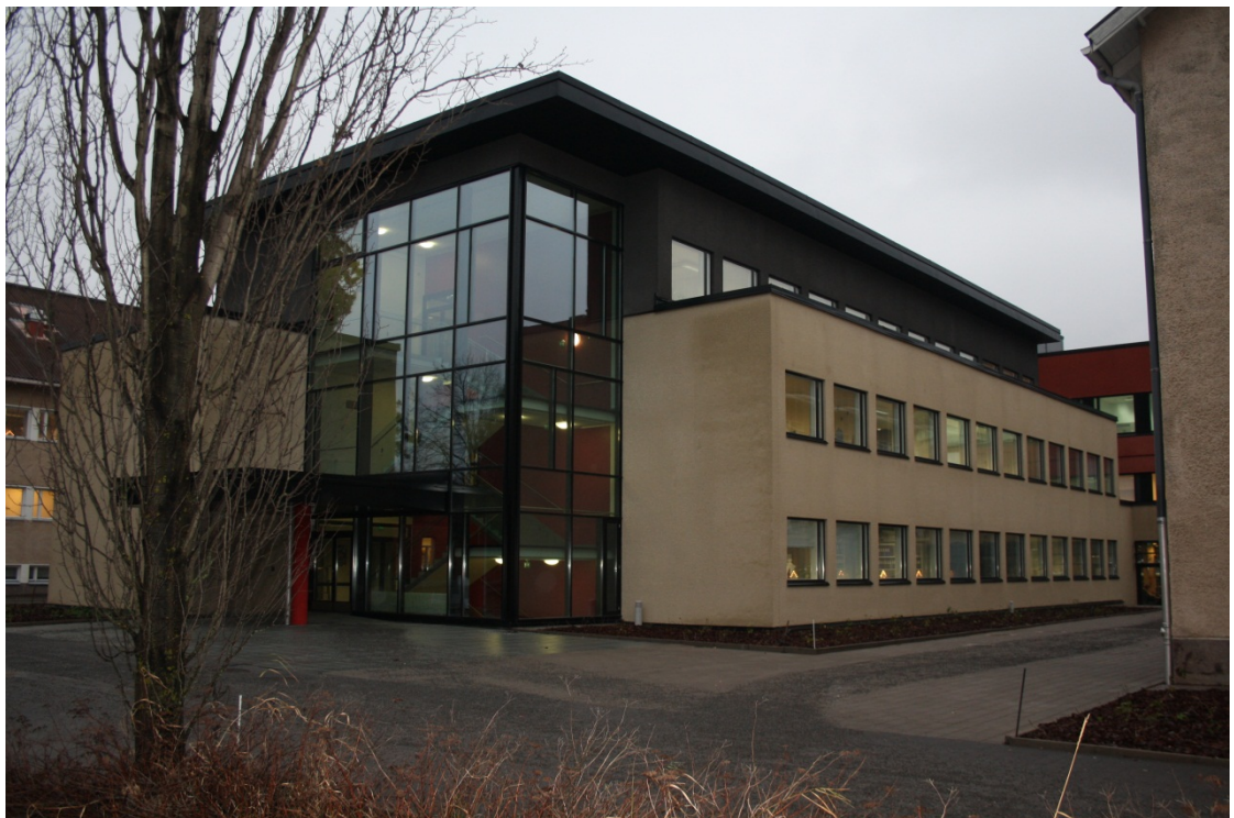
Figure 38. Office building (case 3).
