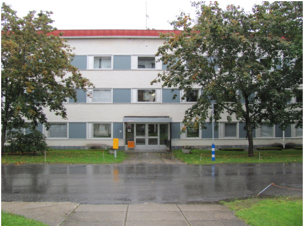
Figure 15. Hospital administrative building.
