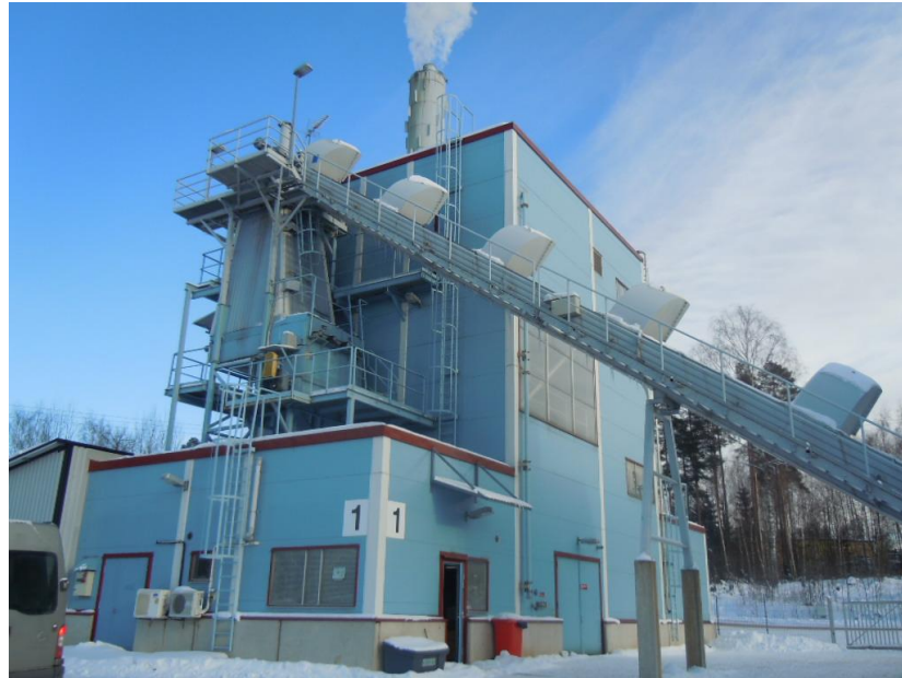
Figure 16 Heating Plant in Karkkila
