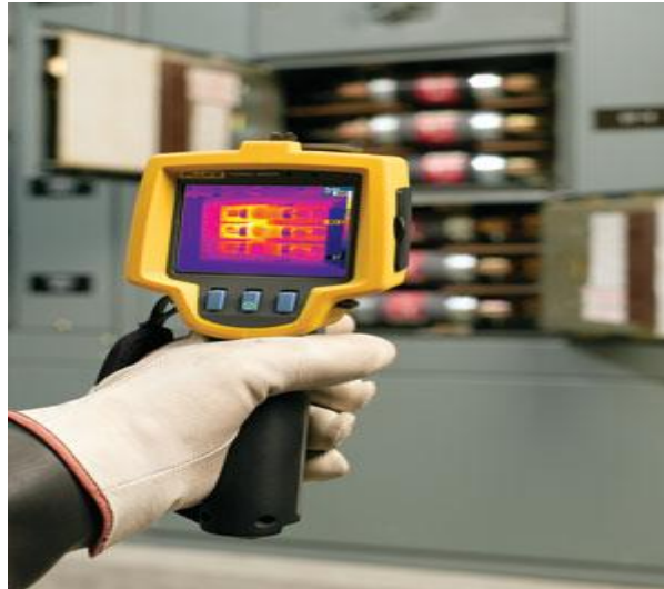
Figure 6 Infrared Termogram made by fluke
