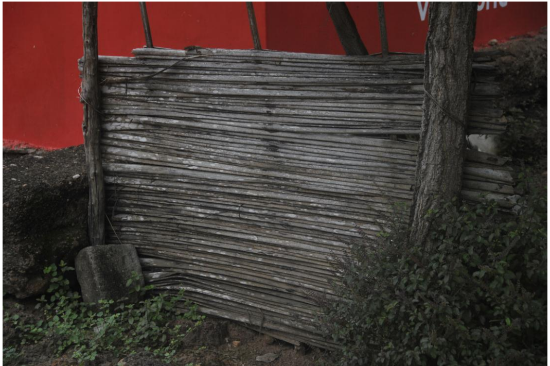
Figure 22. Palm fence that can be used to mark out the limits of the landfill.
