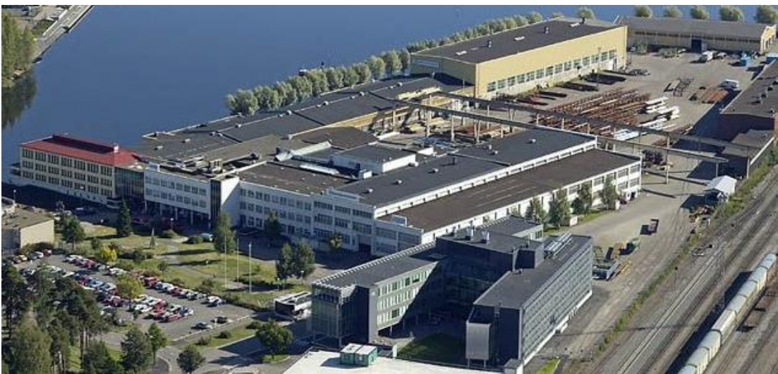
Picture 2. The factory area of Pirtinniemi 2011 (Intranet)
