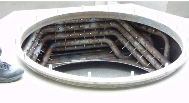
Figure 23. Burner Openings, bended tubes
