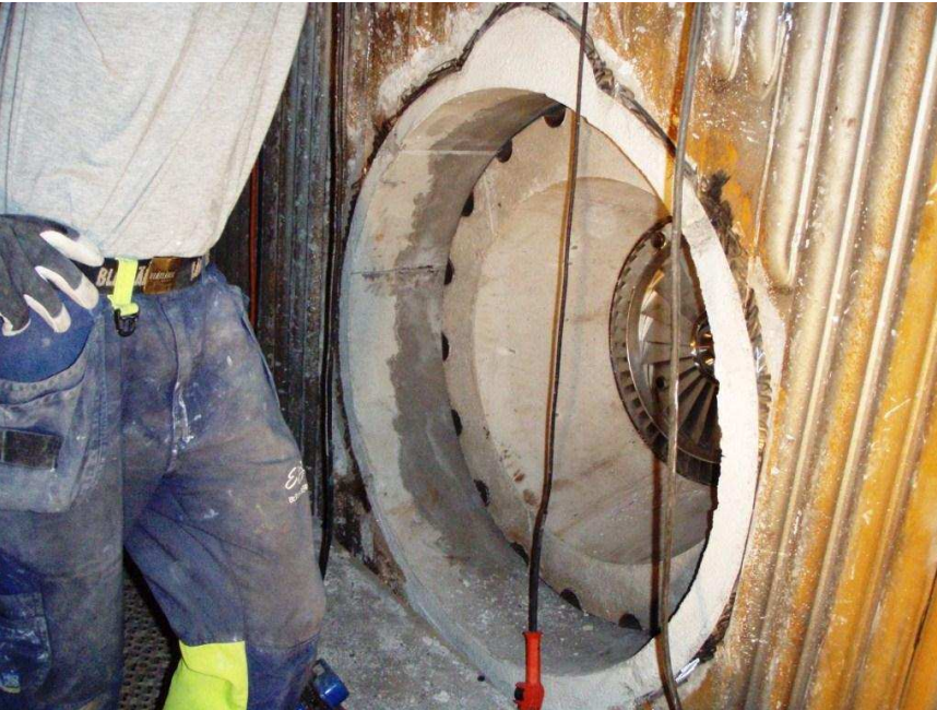
Figure 26. Finalized refractory, seen from inside of the boiler
