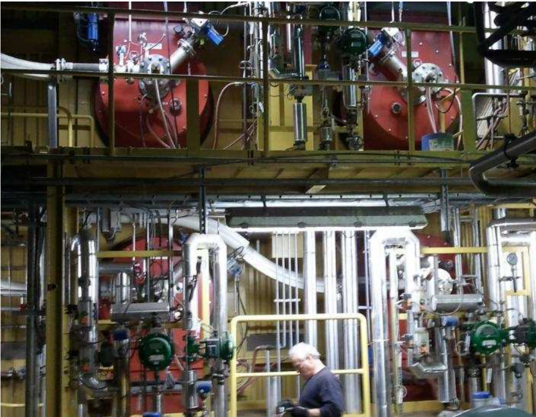
Figure 16. Burners, installed
