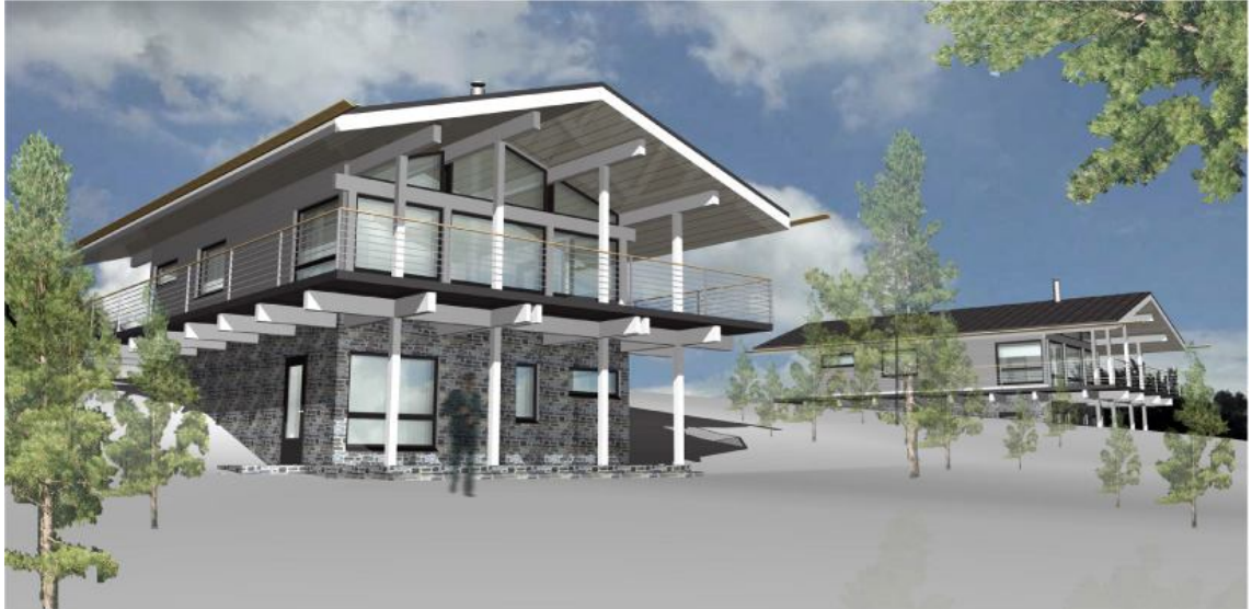
Figure 1.2. Saimaa Villa in Puumala
