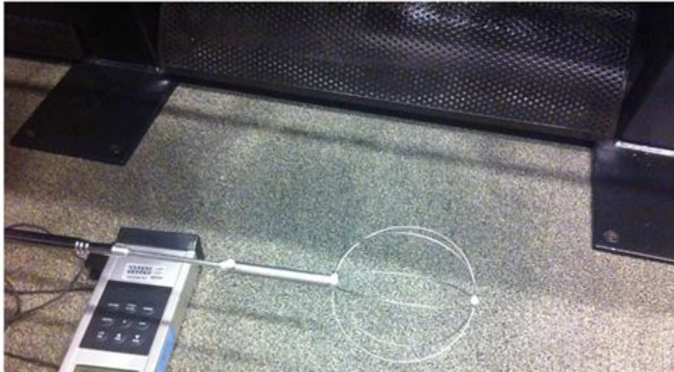
Figure 23. Air velocity measurement of supply diffuser
