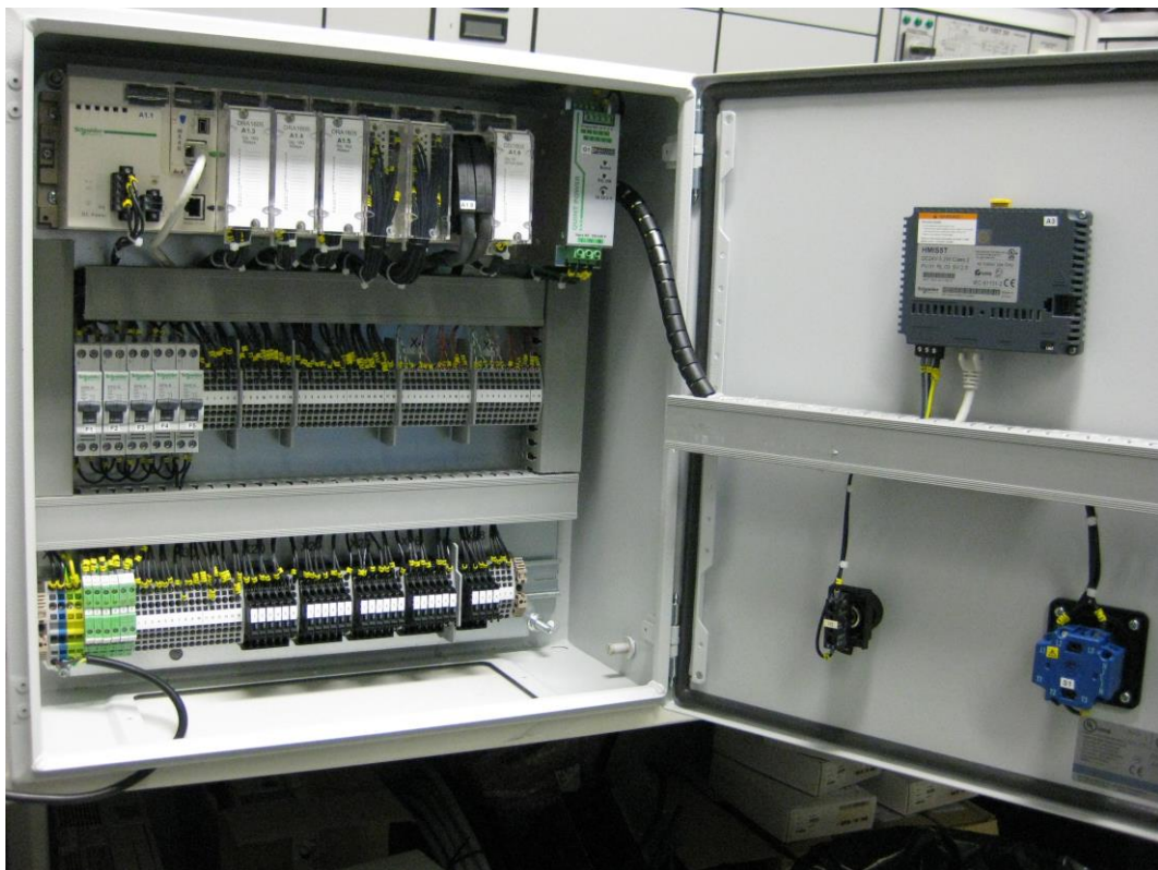
Figure 20. Assembled control cabinet
