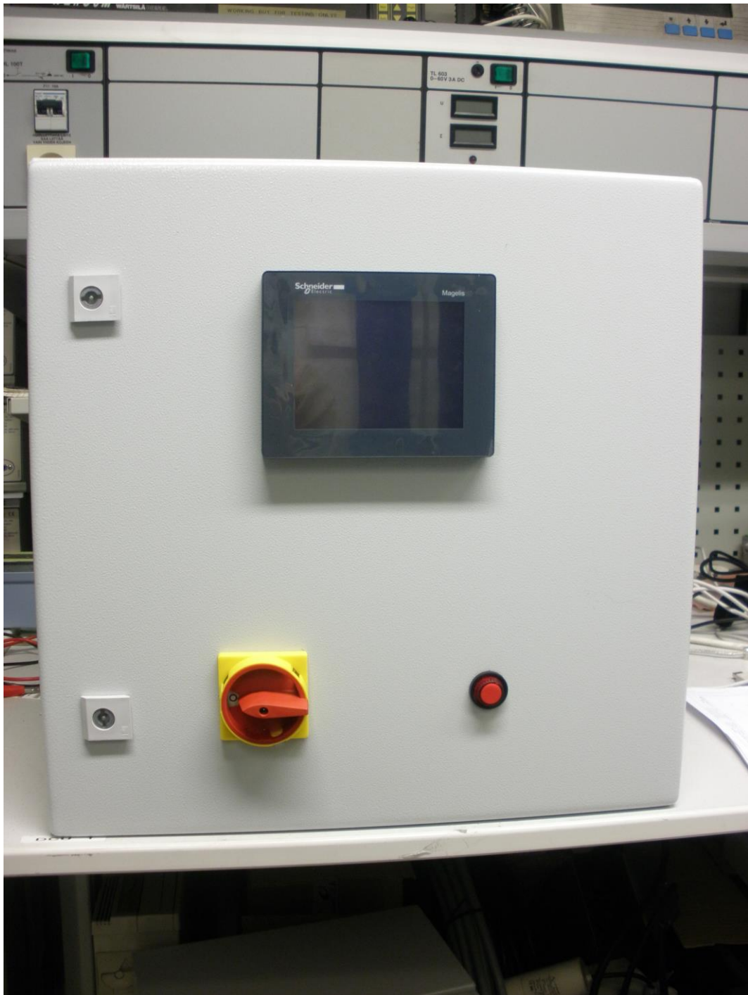
Figure 21. Ready control cabinet
