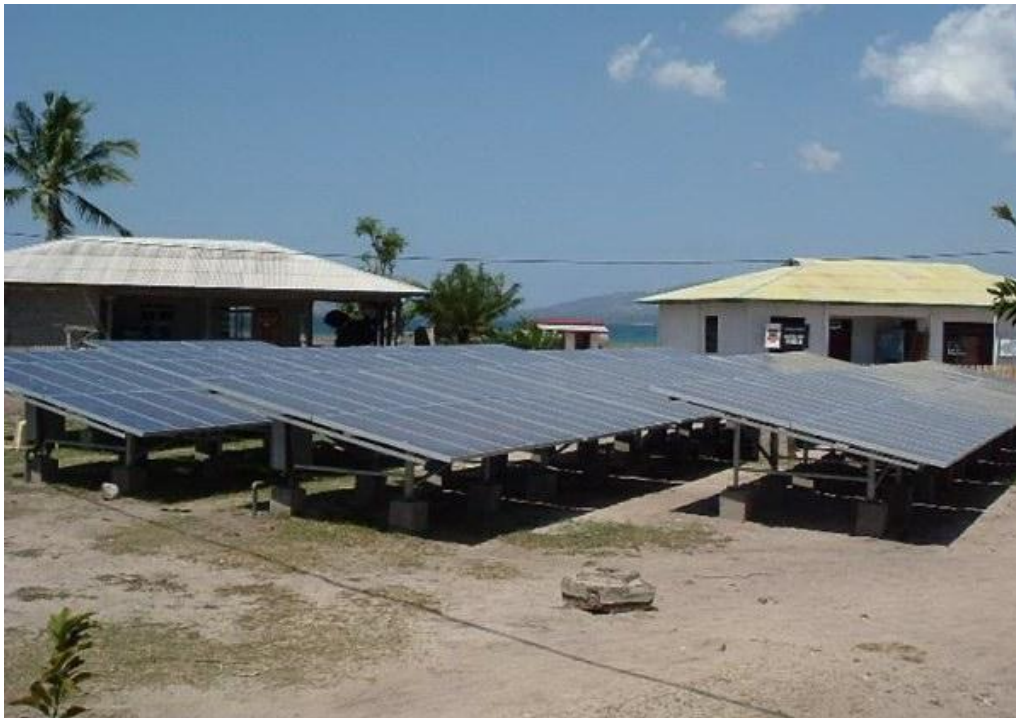
Figure 6. A mini-grid in a rural community comprising 24 KWp PV, 20KWh battery and 125 KVA genset. Photo adapted from Transenergie [40].
