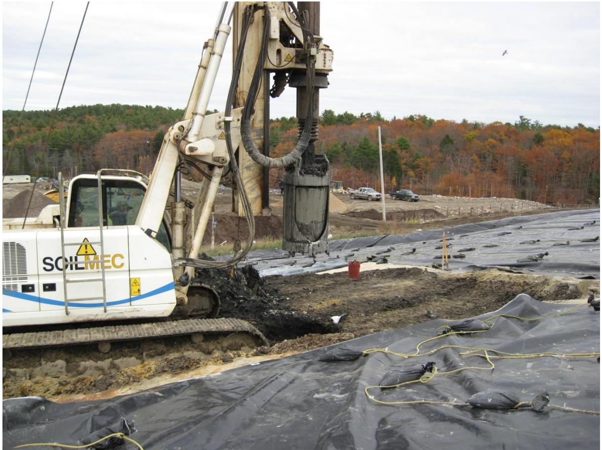
Figure 6: Drilling equipment for a gas well and installation of the gas pipe
