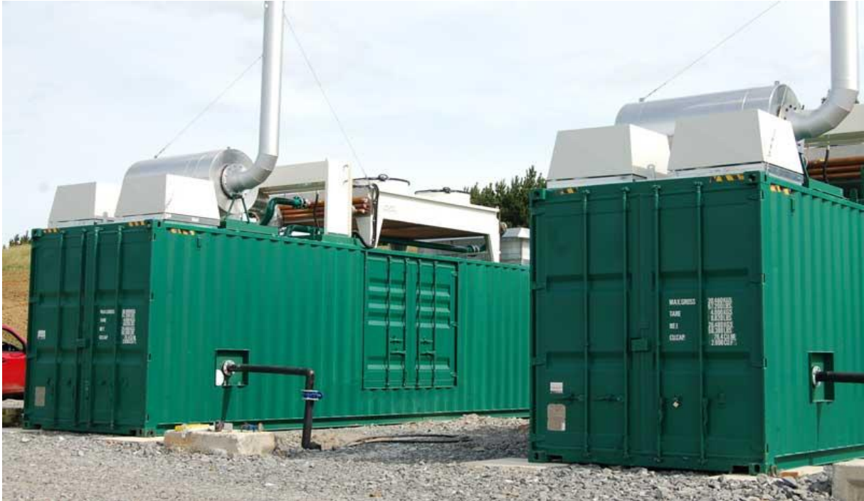
Figure 9: Connection of gas pipes to a pump and regulation container
