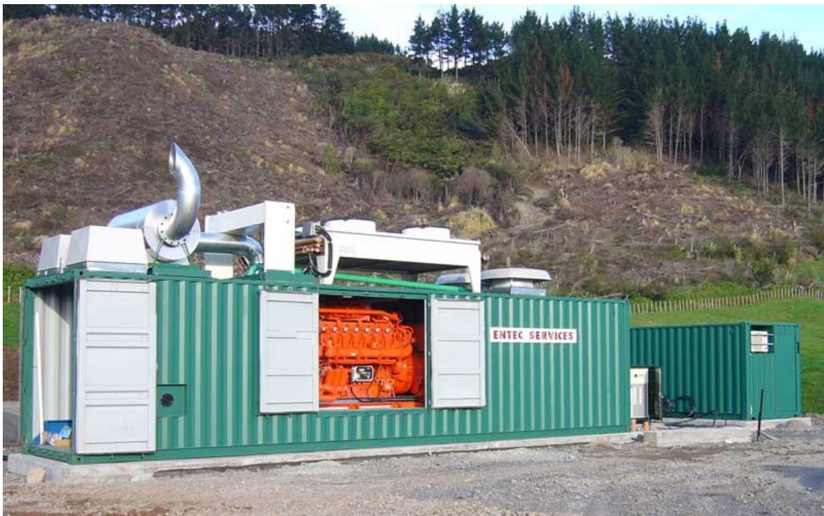
Figure 8: Installing of a container with a compressor and gas cooling system
