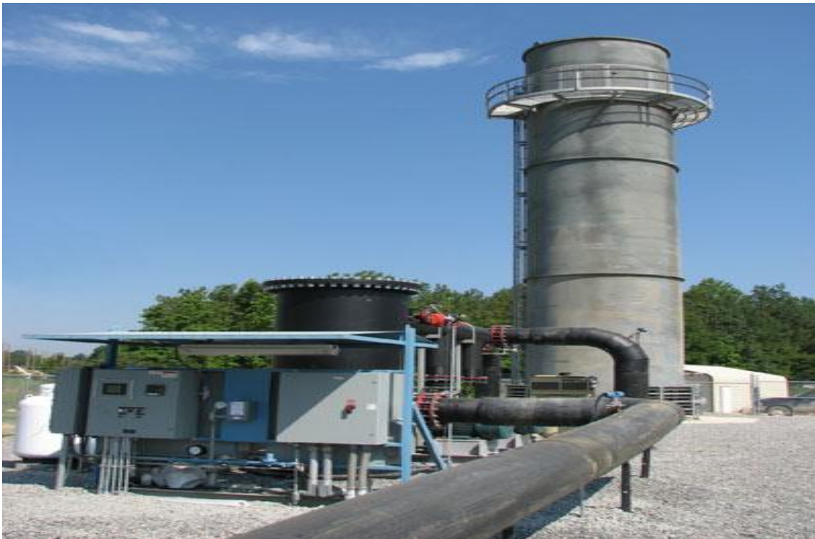
Figure 10: Measuring equipment on an enclosed flare
