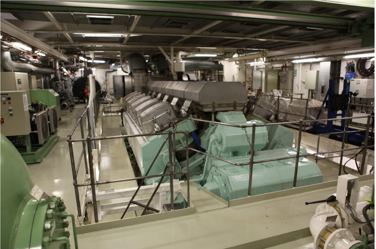
Figure 8. Main engine room. (Kenneth Karsten)
