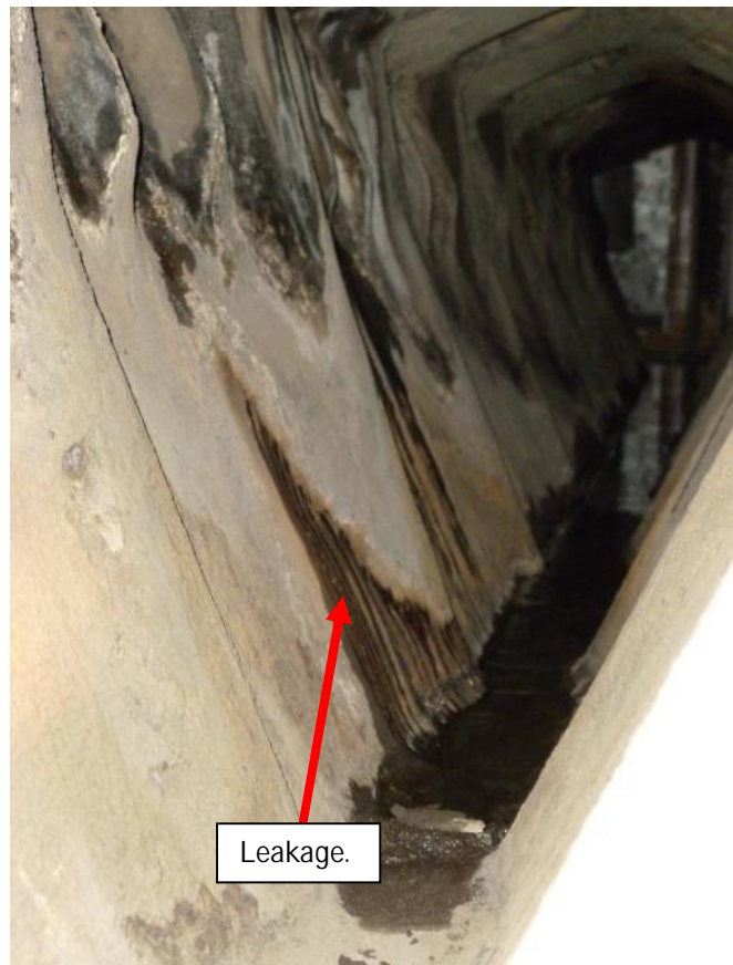
Figure 34. Leaking repair.
