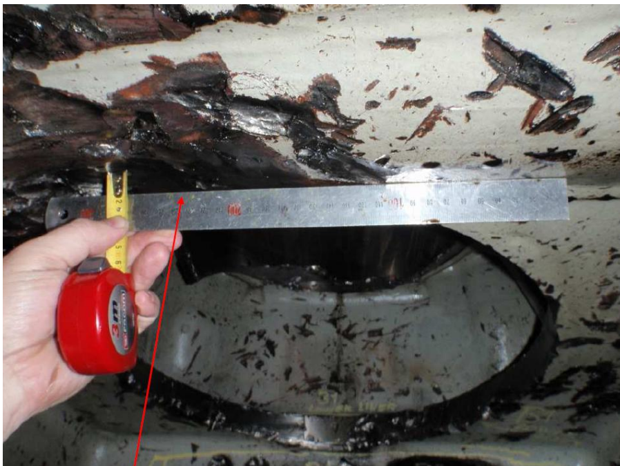
Figure 41. Damaged HT-water channel.
