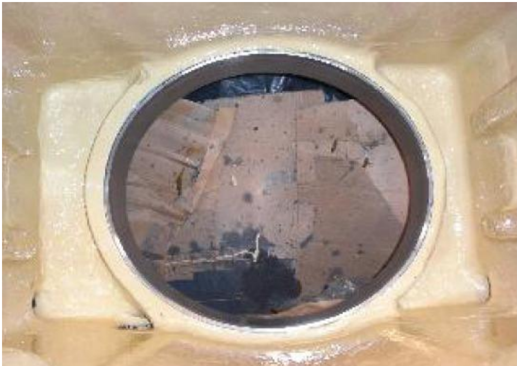
Figure 22. Job finished and ready for pressure testing.
