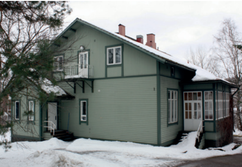
Wolmar Forsberg designed to Koskenranta a residential house which is one of the oldest in the area.
