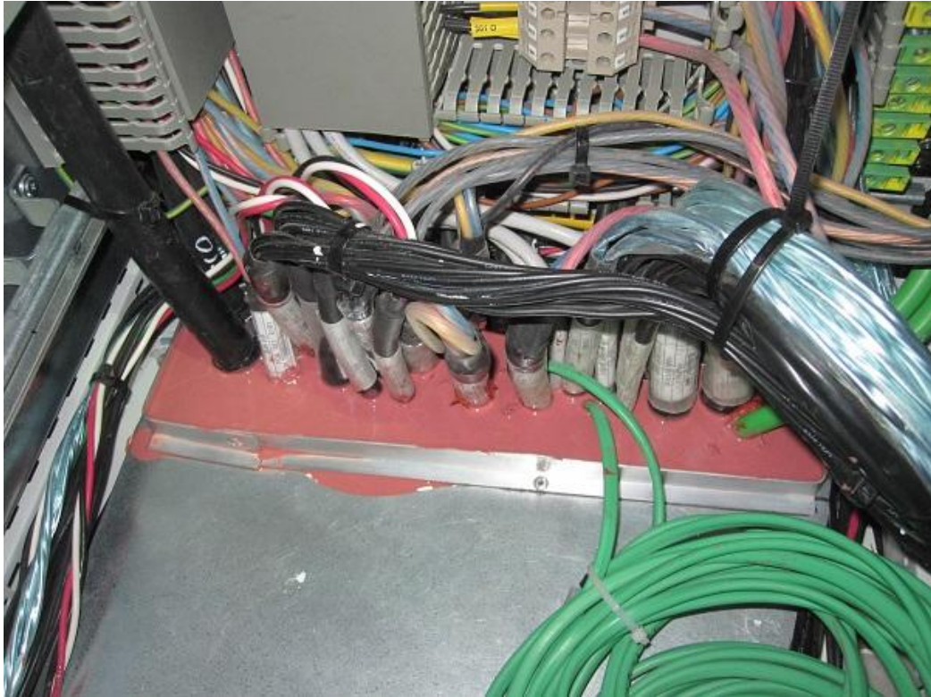
Figure 22. The Elastasil compound has been poured into surrounded area /21/
