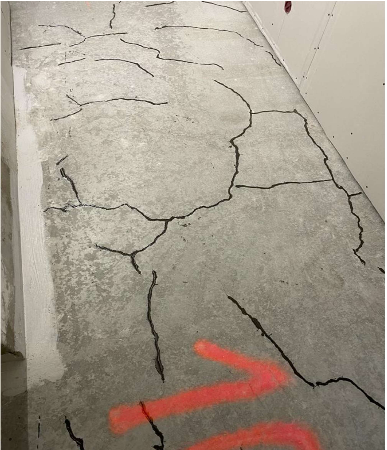
Figure 12 shows injected slab
