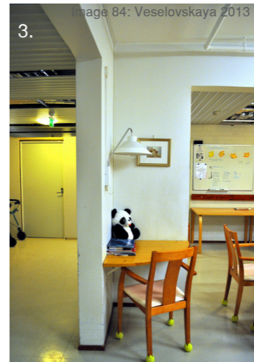
3. L-shaped load-bearing wall, dining room
