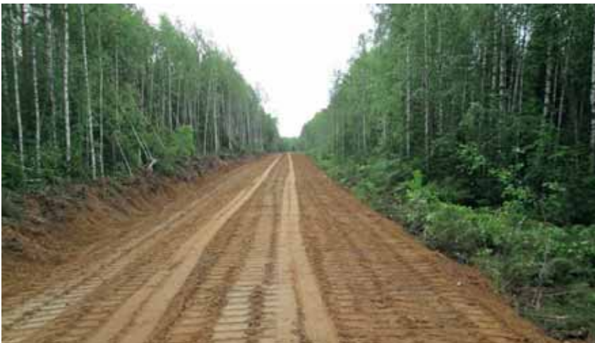
PICTURE 4. A finished base for a forest road in Perm (Laiho).
