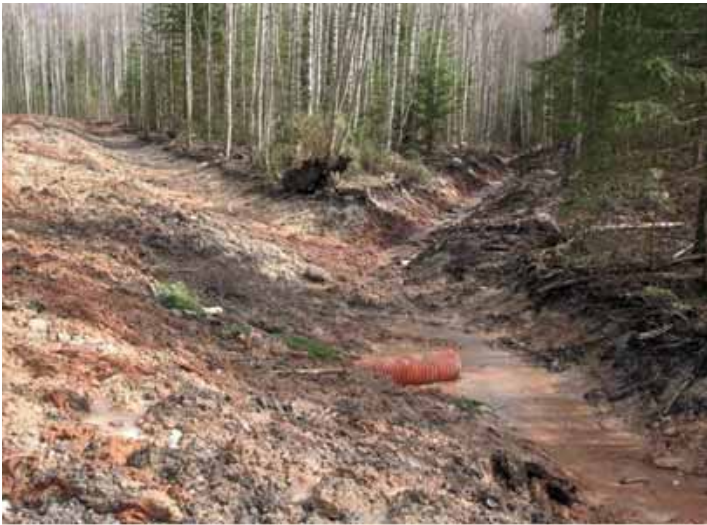
PICTURE 3. Drainage of a road body in Tikhvin (Greis).
