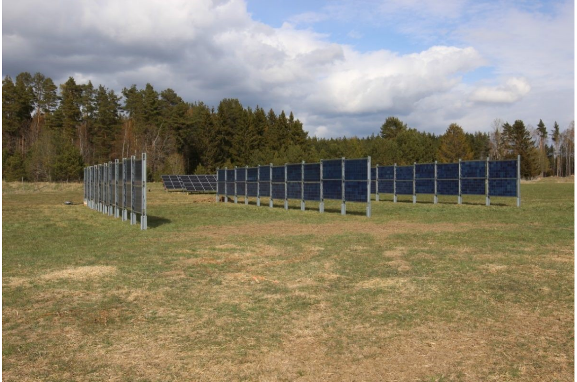
Figure 7. Agrivoltaic research site at Västerås, Sweden (Bellini 2021).
