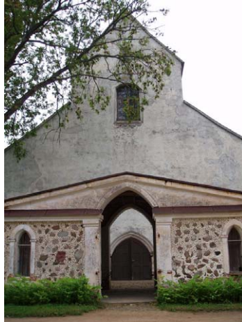
Figure 10 Church with the arch in Rujiena. (Photo: Mari Viskari, 2005)
