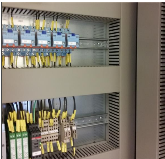
Figure 4. DIN rails with components mounted on the mounting plate.
