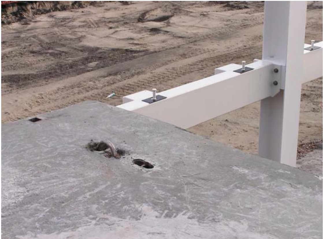
PICTURE 6. Detail of parking garage (IFD Bouwen 2014)
