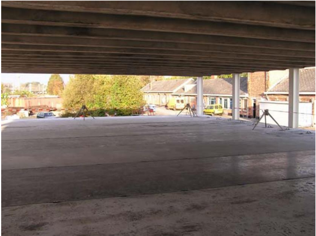
PICTURE 7. Overview of parking garage (IFD Bouwen 2014)
