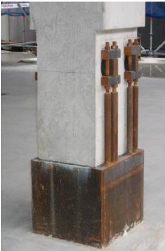
PICTURE 4. Detail of foundation
