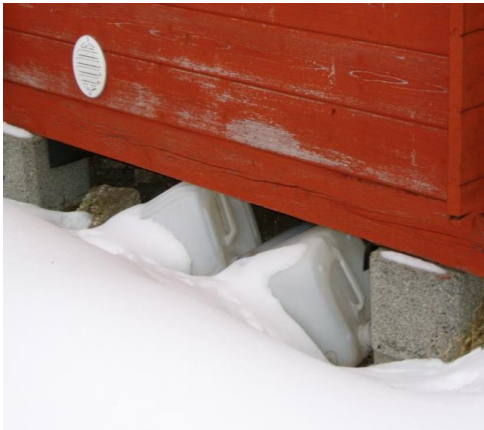
Photograph 2 Canisters in which the dry toilet leachate is directed
