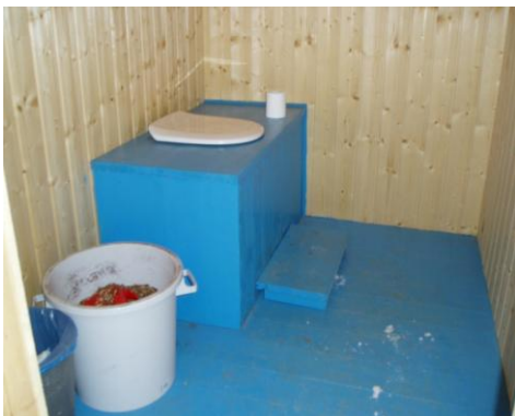
Photograph 3 A Nekala dry toilet from inside
