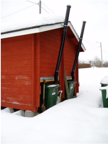
Photograph 1 A dry toilet from Nekala with the Green Toilet 330 and ventilation pipe in sight
