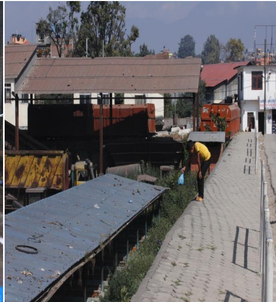
Improper waste disposing
