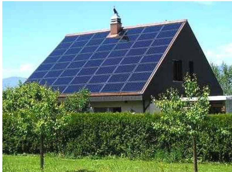
Figure 4: Building with solar pannels on the roof
