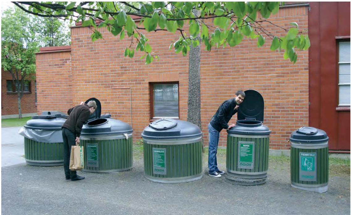
Figure 8: picture showing an underground household sorting bin (Piippo 2013, 1).
