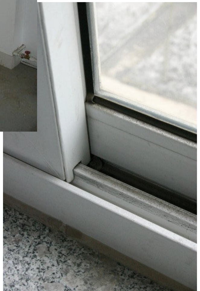
Picture4- 7, window structure
