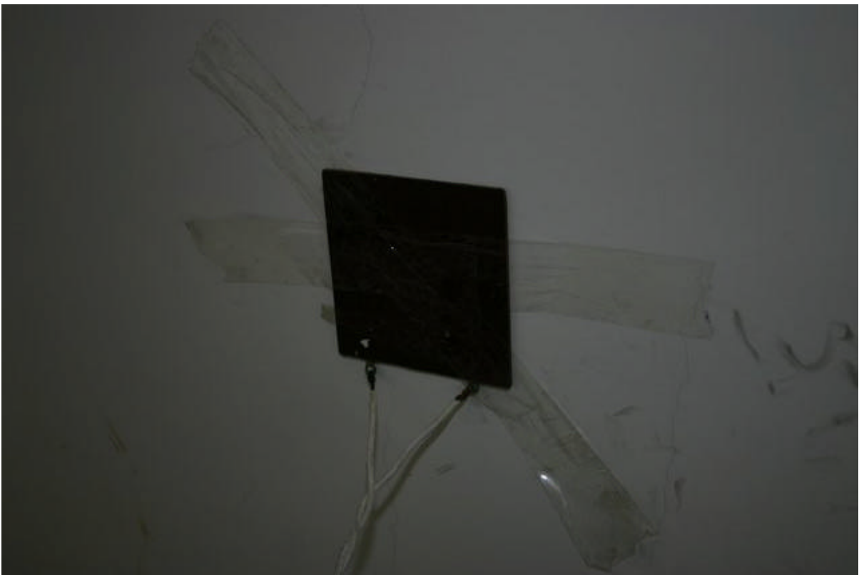
Picture 4-3, Heat flow sensor on the outer wall.
