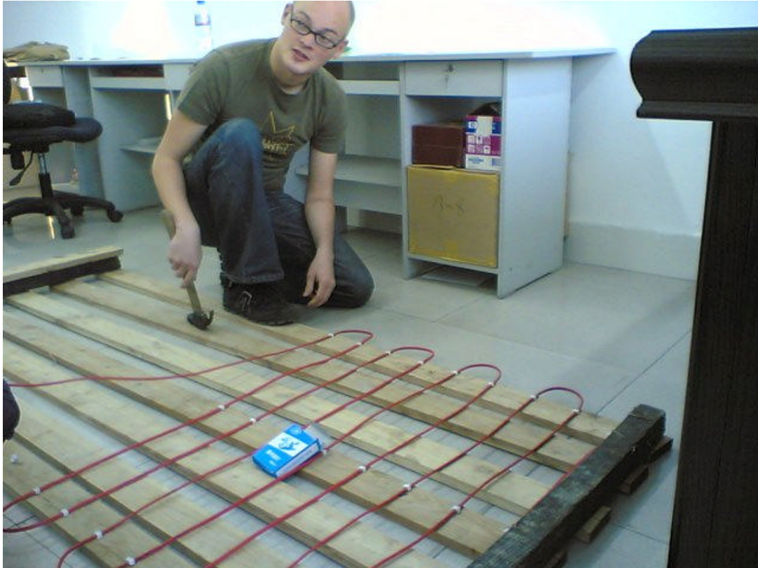
Picture 4-8, Building the bed (2 wire system)
