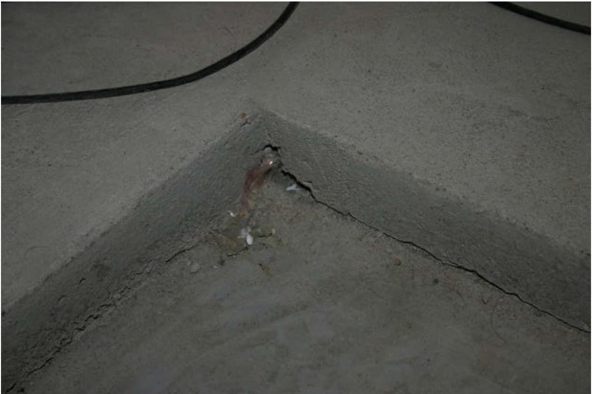
Picture4- 5, afterwards constructed floor structure (taken from the door)
