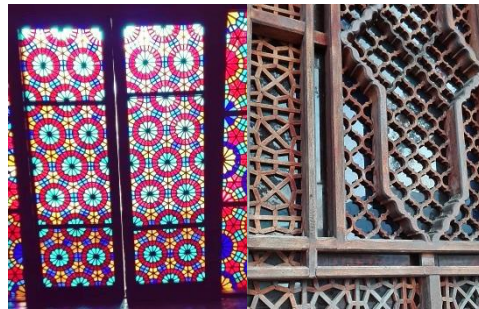
Picture 4 Shaki Khan's Palace's Shabaka window from outside and inside in Sheki. utilized instead of ordinary doors and
