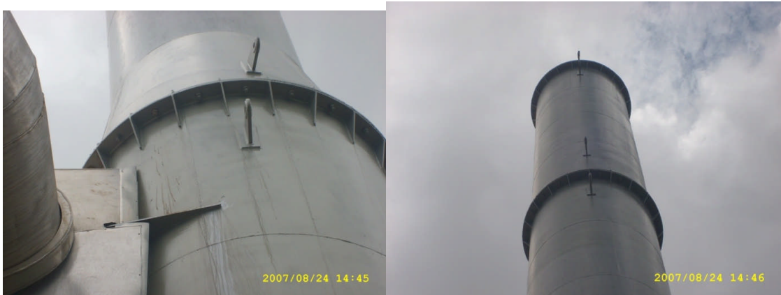
PICTURE 6 & 7. Stack duct & industrial chimney constructed for Nestle by the C.E.O. (Photos: Femi Adefolalu 2007)
