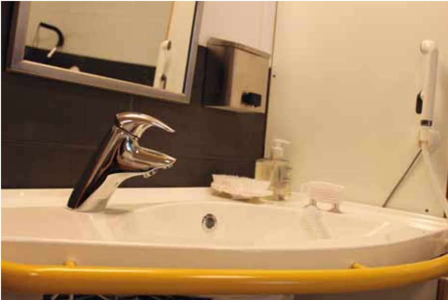
Figure 8. The height of the sink can be adjusted, contrasts help perceive things more clearly (Photo: Ronan Browne)
