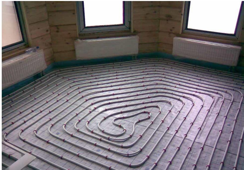
Figure 20. Water floor heating system
