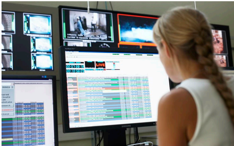
Picture 1. Master control room operation [Levira Ltd]
