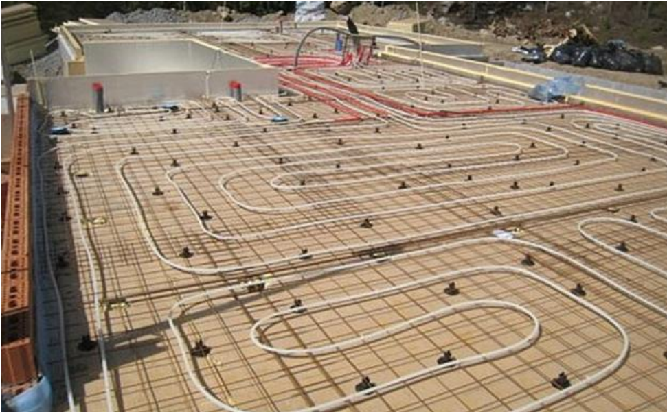
Figure33: Ground floor heating structure.
