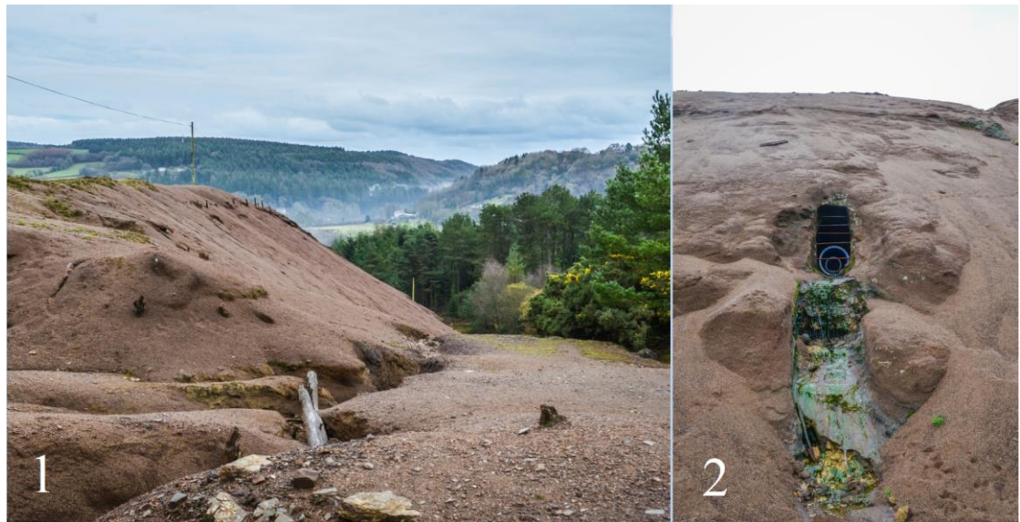
Figure 2. Erosion and leachate at the DGC. Source: Author, 2014
