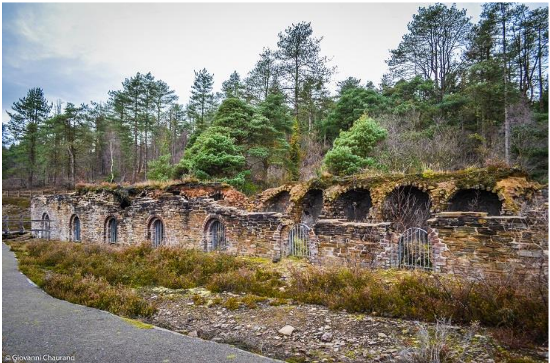
Figure 4. The remains of the labyrinth condenser at DGC. Source: Author, 2014
